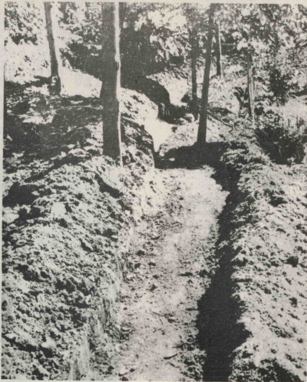
The first step in making a contour mound is to dig a trench.
