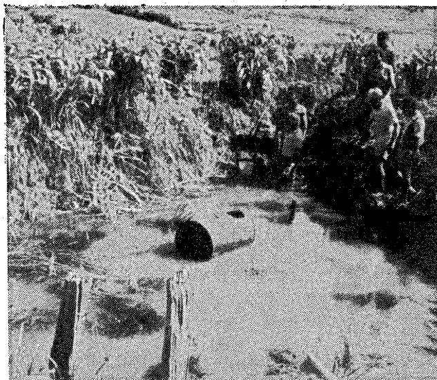
The water system at Koroba - the pond has just been drained. Note the vegetation growing at the sides to make the walls stronger.
