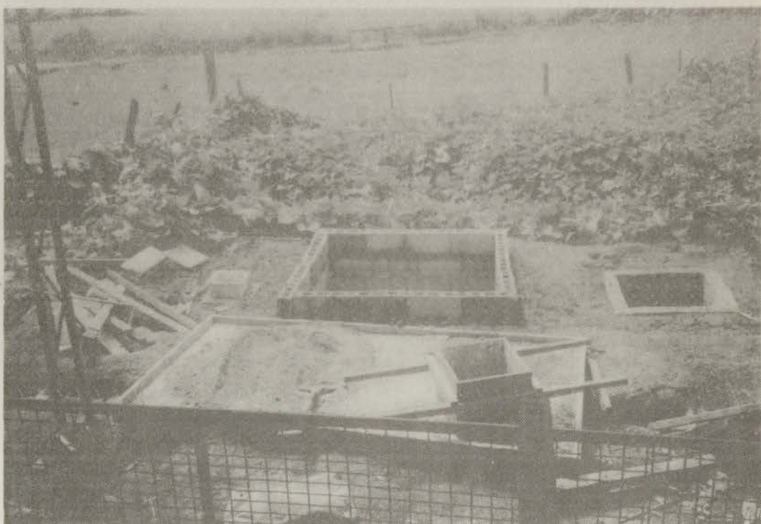
Cementing of the floor of fermentation tank
