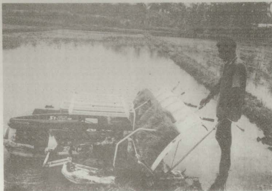
Figure 8. Seedlings from the nursery boxes can be mounted onto a mechanised transplanter for transplanting in the paddy field.
