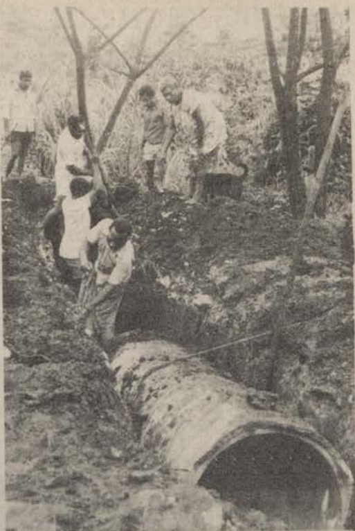
Mrs Wirua supervising the placement of a culvert under the road at Babata.
