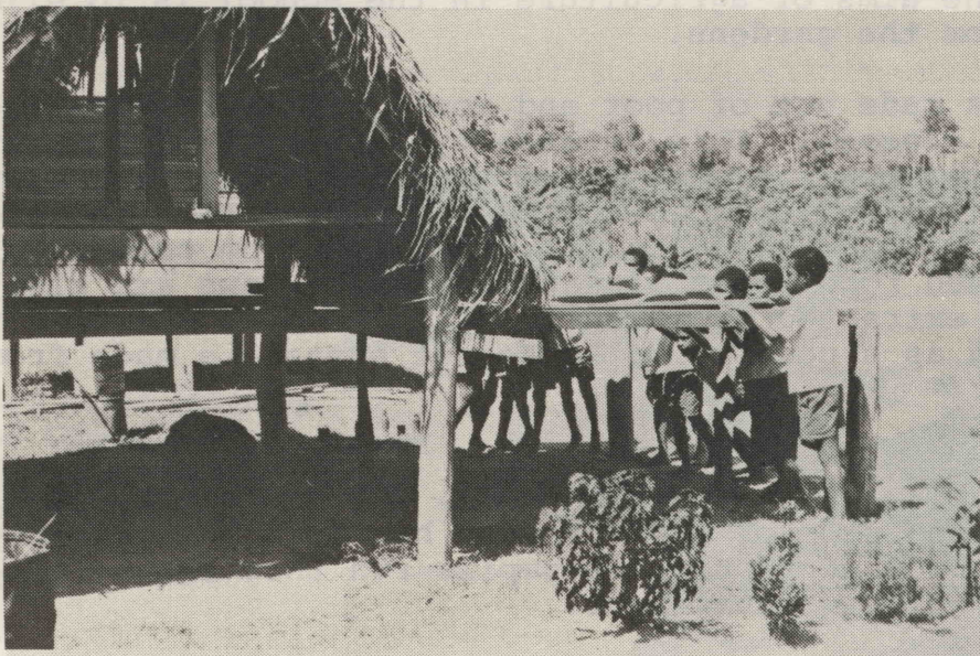
The drying house which has a sliding floor which can be slipped in and out depending on the weather
