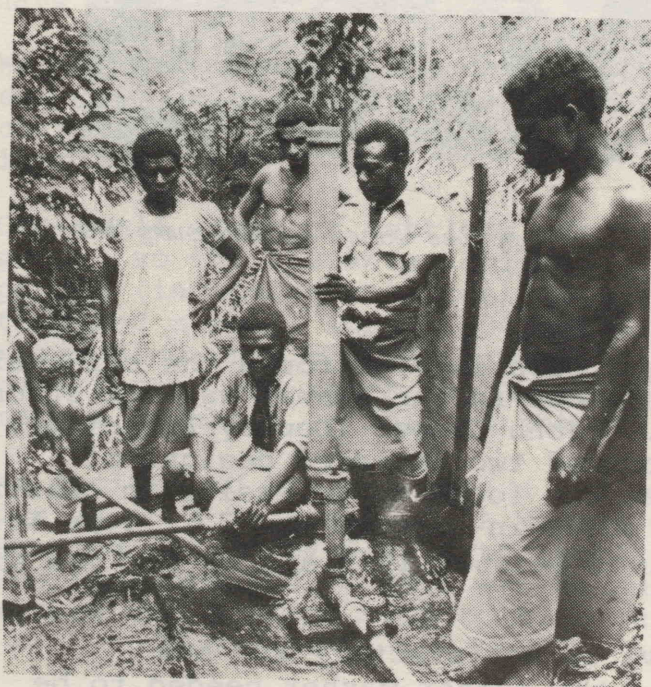
Turning on the pump. Note the drive pipe on the right which comes from the dam and the delivery pipe on the left which goes up to the village
