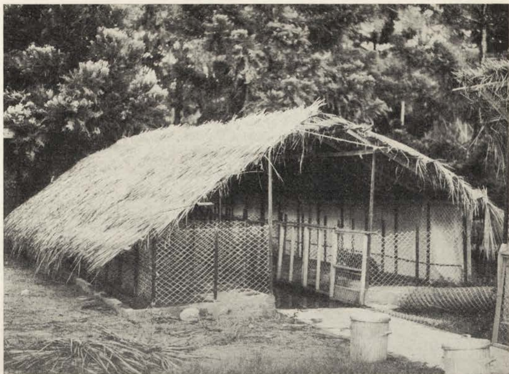
Plate II.—Pig house with bush material walls and roof, and concrete floor
