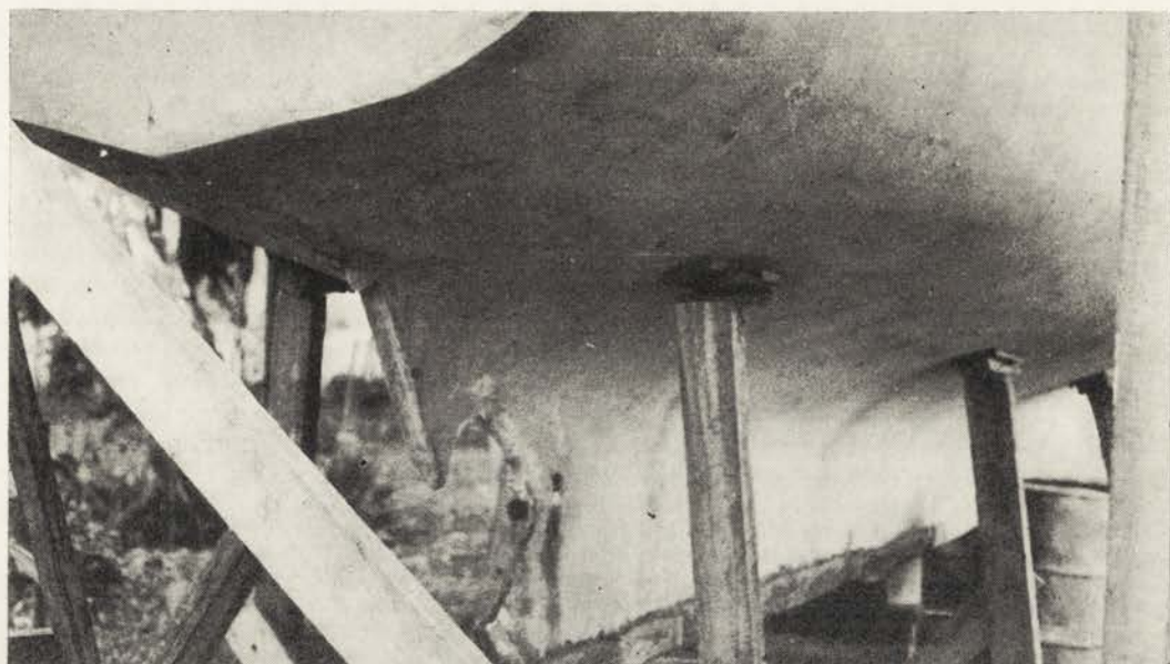
Plate V.—A close-up of the hull before being painted, showing the smooth finish of the cement
