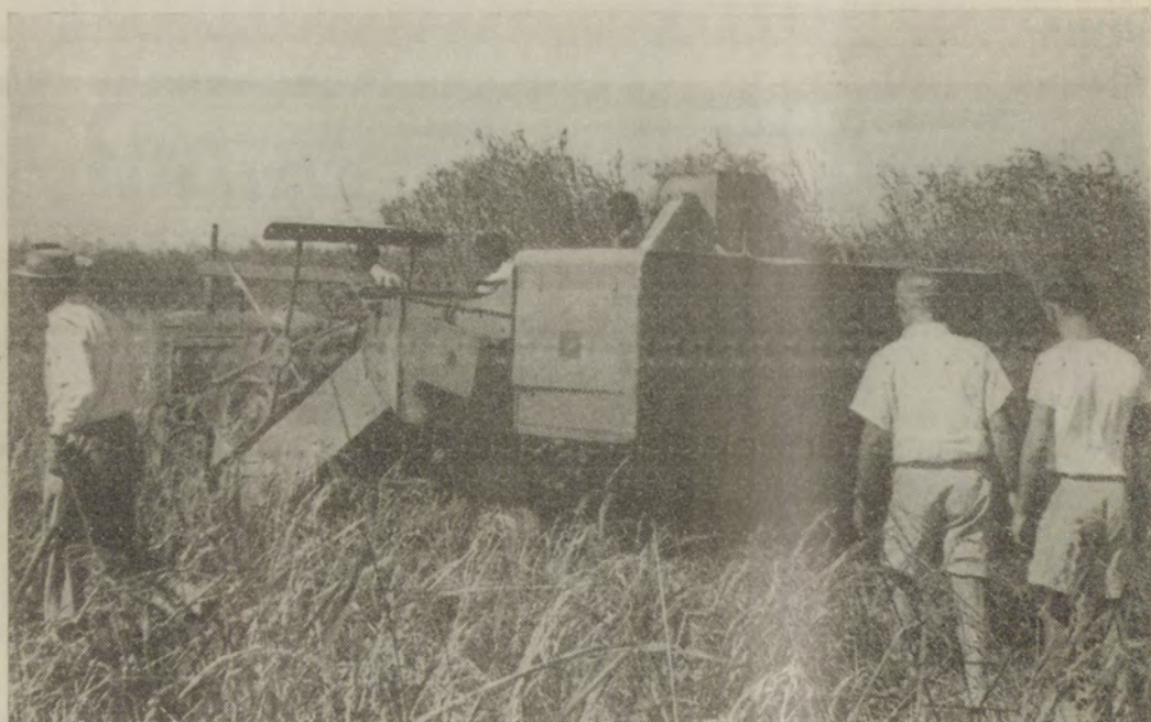
Fig. 4.—Harvesting a partially lodged rice crop in the Mekeo area using an open-front header.
