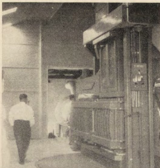
Plate XII.—The automatic hydraulic baling press.
