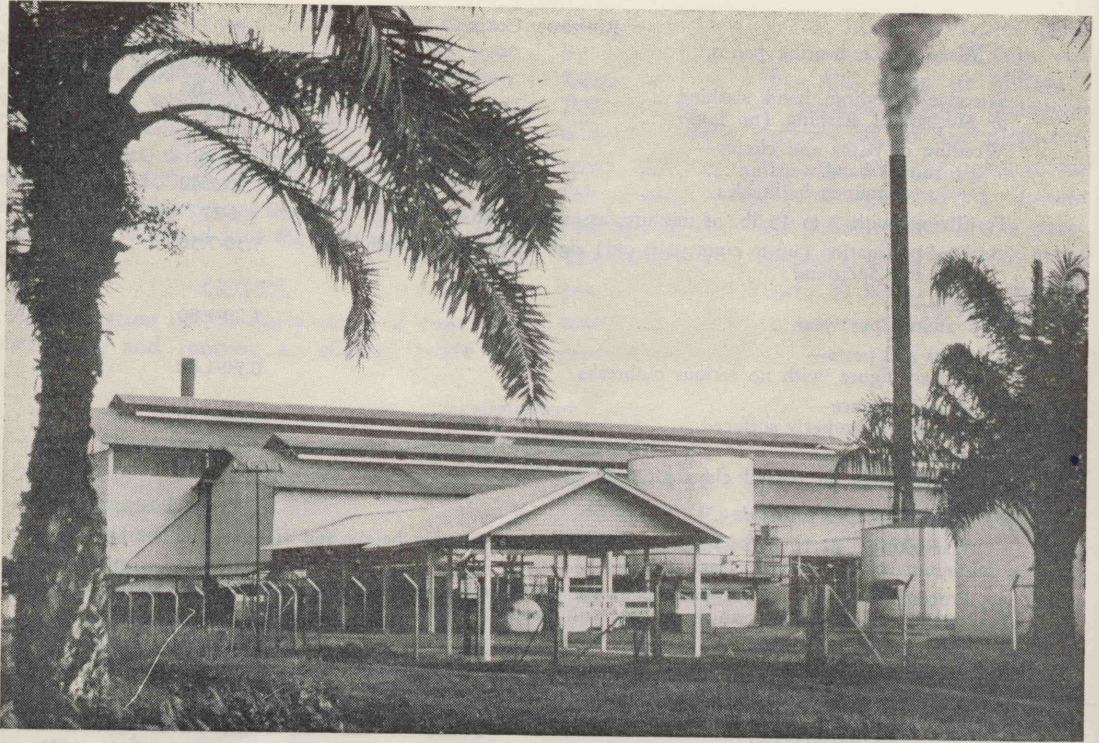
Plate XIII.—A typical oil mill. The weighbridge is in the foreground, with the horizontal sterilizers directly behind. To the right are bulk oil storage tanks.
