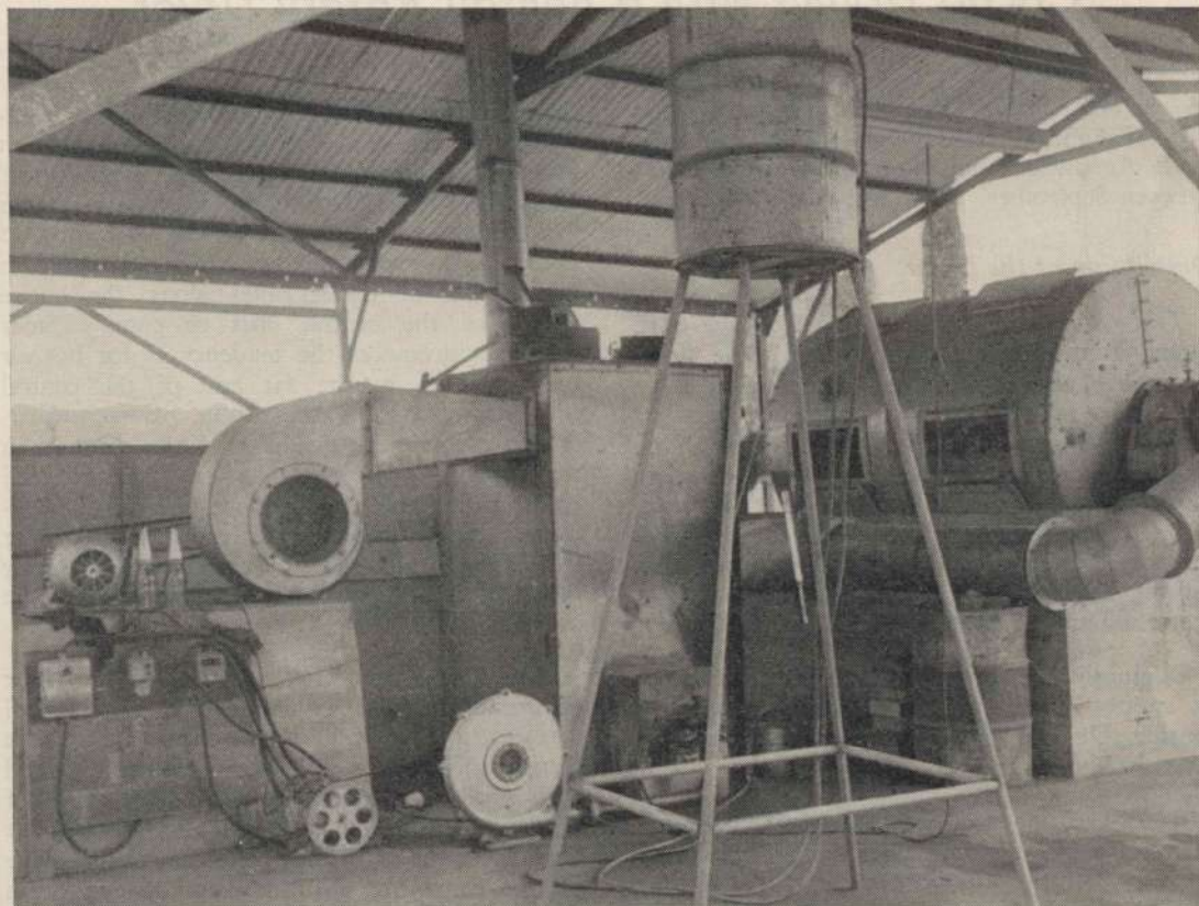
Plate I. —A general view of the dryer with fan and heat exchange unit.
