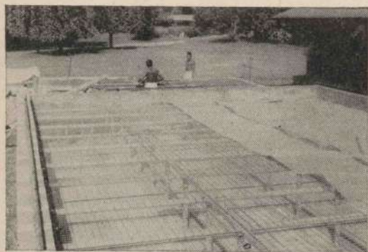
Plates I and II. —Details of construction showing steel pipe framework supporting A.R.C. mesh and cocoa wire drying floor. Note steel bolts set in concrete around the edge of the floor to take the 3 in. x 2 in. framework and marine plywood facing board.
